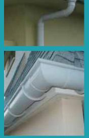
Fit Downpipe brackets at 2 metre spacings for vertical pipes and 1.2 metres for graded pipes.
